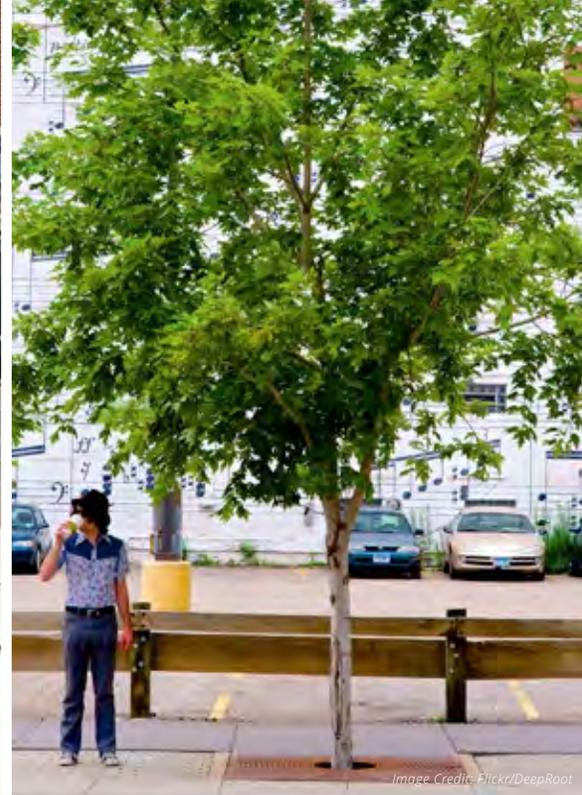
A stormwater tree is a street tree planted within soil that is lower than street level to capture stormwater from roads and sidewalks. The tree absorbs stormwater through its roots. Some stormwater tree pits have metal grates above them. Others have inlets that direct stormwater to the trees.
