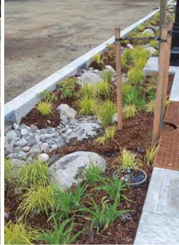
Green gutters are continuous, narrow areas with soil and plants that are put along the edge of a street where it meets a sidewalk, with a new curb at the street edge. The soil and plants are lower than street level to capture stormwater from roads and sidewalks. Green gutters can vary in size and materials.
