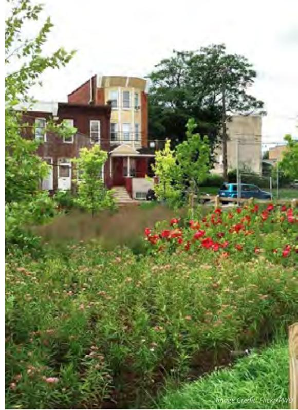
A rain garden is an area with soil and plants that is not surrounded by a curb. Rain gardens are typically located in grassy areas. The soil and plants are lower than surrounding areas to capture stormwater. The stormwater collects in the rain garden, creating a small, shallow pond until the water drains down through the soil. Some rain gardens have an underground storage system beneath them to hold more stormwater. Rain gardens can vary in size and materials.
