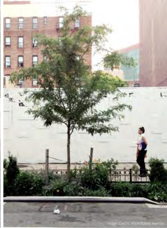
A stormwater planter is an area with soil and plants surrounded by a curb, typically located at the edge of a sidewalk where it meets a street. The soil and plants are lower than street level to capture stormwater from roads and sidewalks. Stormwater planters can vary in size and materials.
