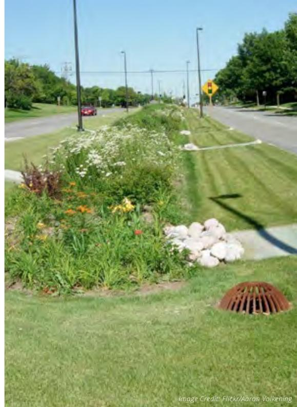
A bioswale is a long, shallow depression designed to slow the flow of stormwater and allow it to drain into the soil. Swales can be used as an alternative to traditional ditches or as a way to slow stormwater before it gets to other GSI.
