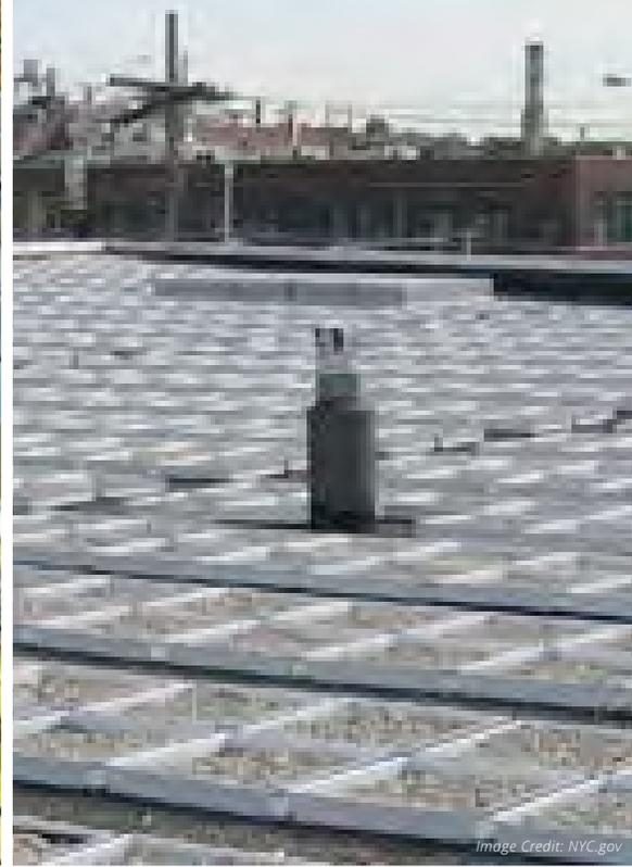
A blue roof is a roof that is either partially or fully covered by a system of stone storage trays. The storage trays capture rainwater until it evaporates. Blue roofs vary in size and can be used alongside green roofs.
