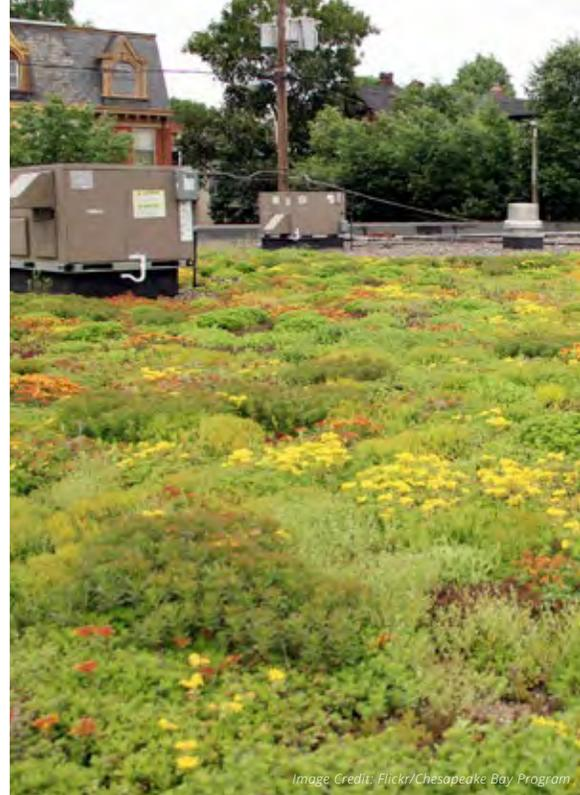
A green roof (or vegetated roof) is a roof that is either partially or fully covered by a system of plants. The plants are put on top of soil or a water storage system. Green roofs vary in size and depth depending on the weight the existing roof can handle.
