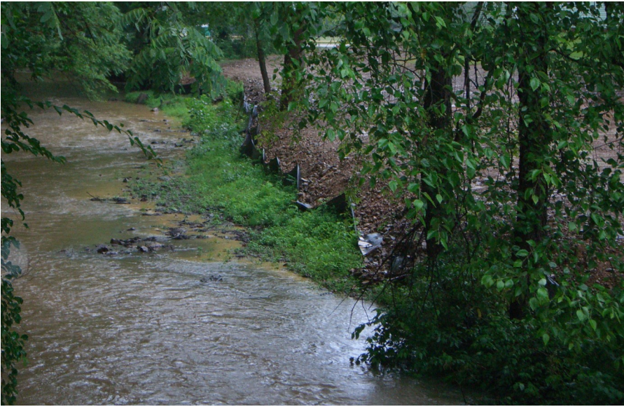
Unattended to Erosion Prevention Measures, June, 2006
