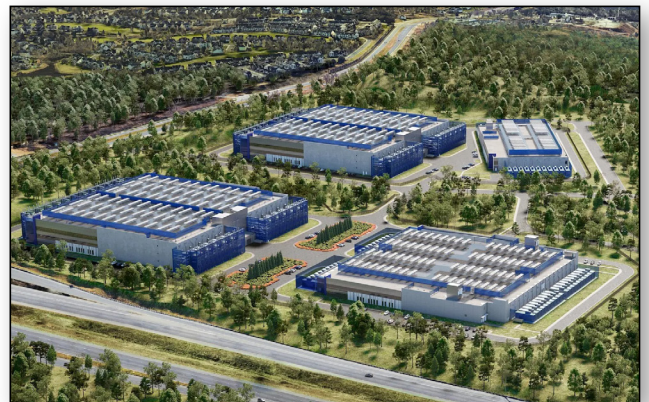
Data center in Ashburn, VA
