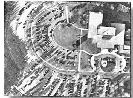
Drone image of Capital Blue Cross parking lot on Elmerston Ave. in Susquehanna Township
