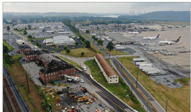
Air Cargo Reconfiguration & Expansion Project at Harrisburg International Airport
