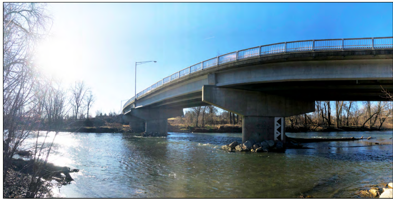
South Hanover Street Bridge at Swatara Creek Park, South Hanover Township
