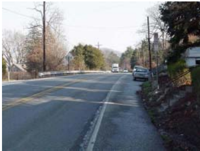
Photo on southbound US Routes 11/15 in the Perdix Area
