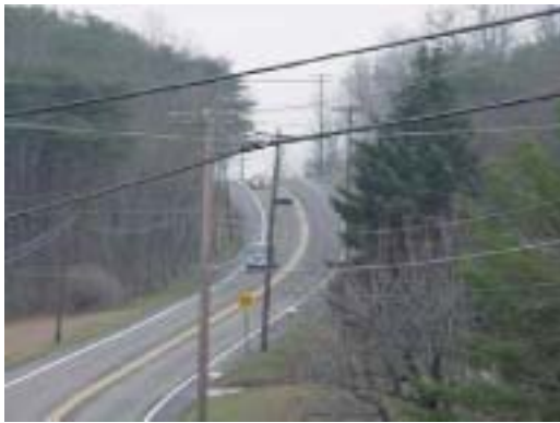
Looking east at the intersection of PA Route 944 and Deer Lane, which is located at the crest of the hill
