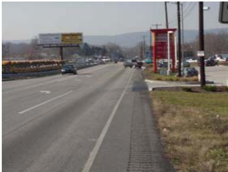
Photo of the view from the northbound approach of US Routes 11/15 looking northbound at the Sheetz / Rohrer Driveway
