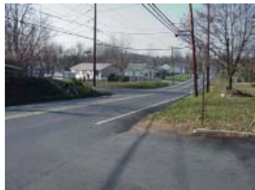
Photo of the offset intersection of PA Route 944 and Magaro Road / Carol Lane
