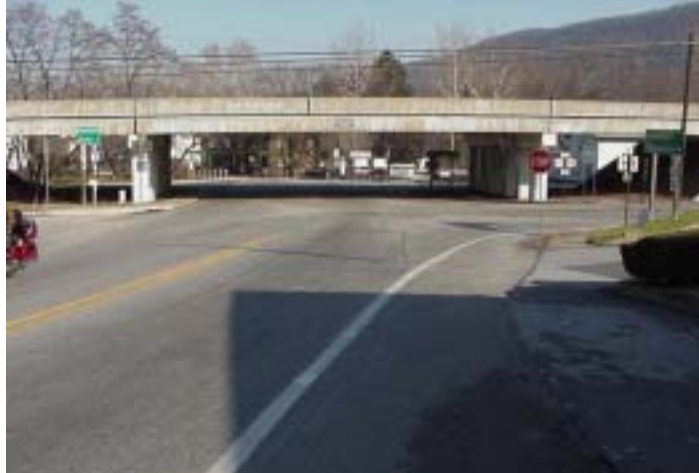
Photo of the view from eastbound PA Route 274 looking at US Routes 11/15 overpass and southbound off -ramp
