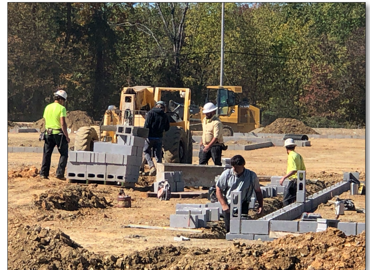
A construction crew at Blue Ridge Village in Lower Paxton Township
