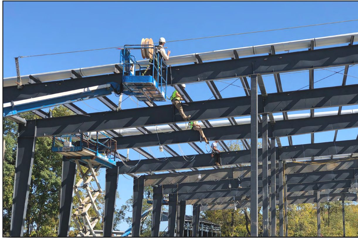
Bloomfield Fire Hall under construction in Perry County
