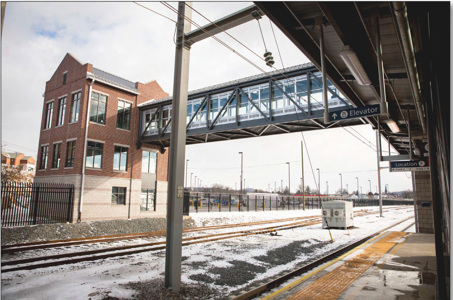
Amtrak train station, Middletown (courtesy Amtrak)
