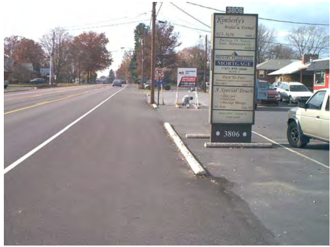
Exhibit 3.29 Curbing with Inadequate Reveal
