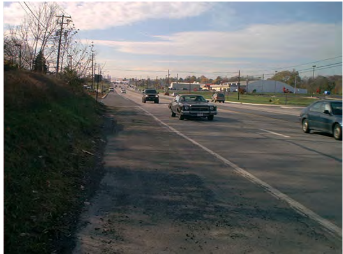
Exhibit 3.28 Deteriorated Shoulder
