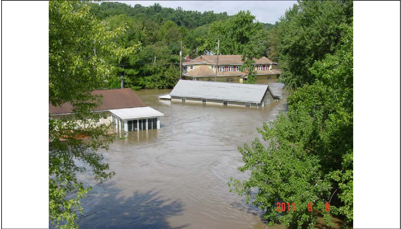
Figure 4.3.2-10 Residential flood impacts in Lower Swatara Township due to Tropical Storm Lee (September 2011) (Lower Swatara Township, 2011).
