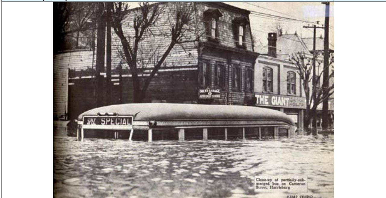
Figure 4.3.2-7 Flooding along Cameron Street in the City of Harrisburg during the 1936 St. Patrick's Day Flood (SRBC).
