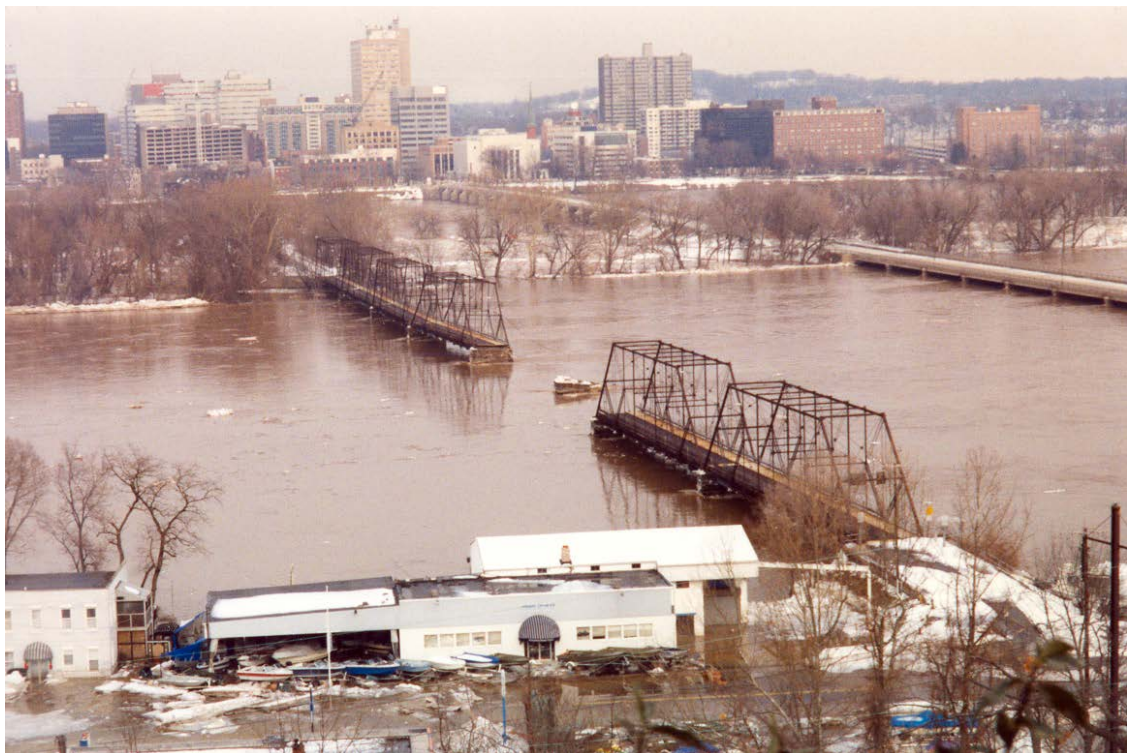
Figure 4.3.2-9 Impact to the Walnut Street Bridge caused by the 1996 Ice Jam Event (SRBC).
