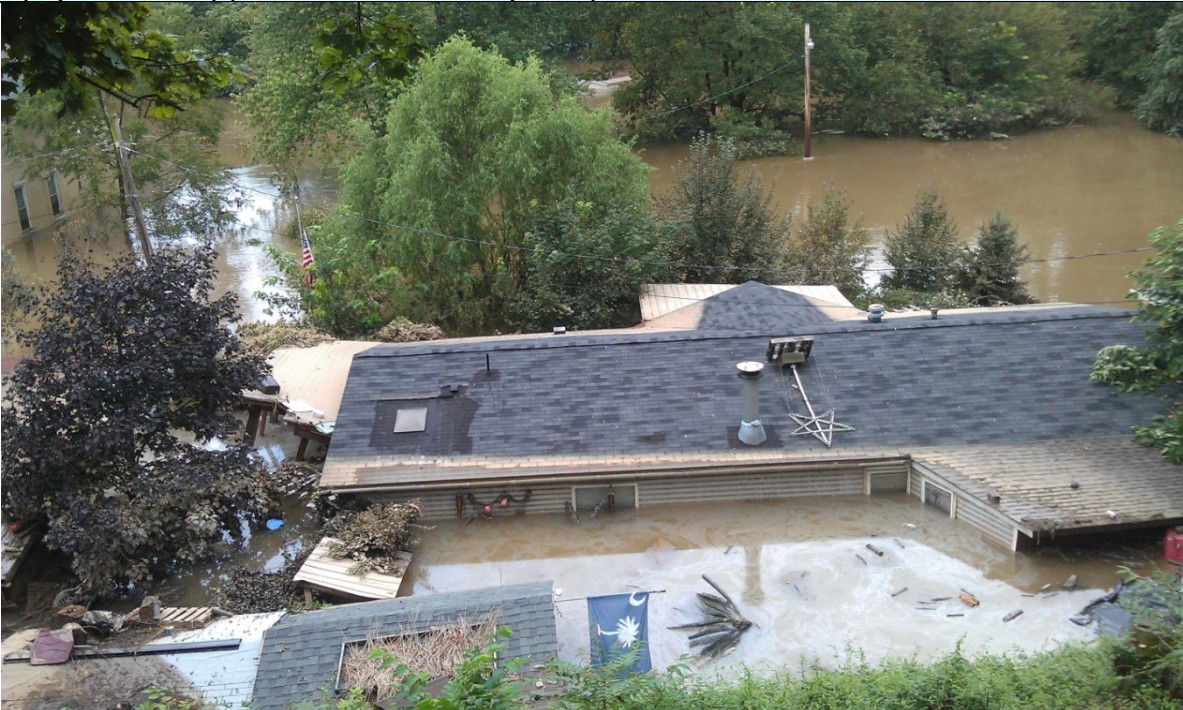
Figure 4.3.2-13 Flooding along Main Street in South Hanover Township due to Tropical Storm Lee (September 2011) (South Hanover Township, 2011).
