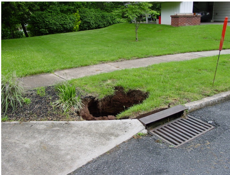
Figure 4.3.7-3 Sinkhole in Lower Swatara Township.
