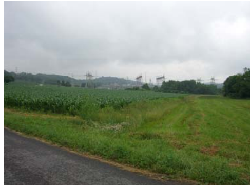
View of PP&L Electric Company's Substation in Centre Township
