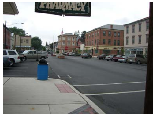
Newport Borough Historic District
